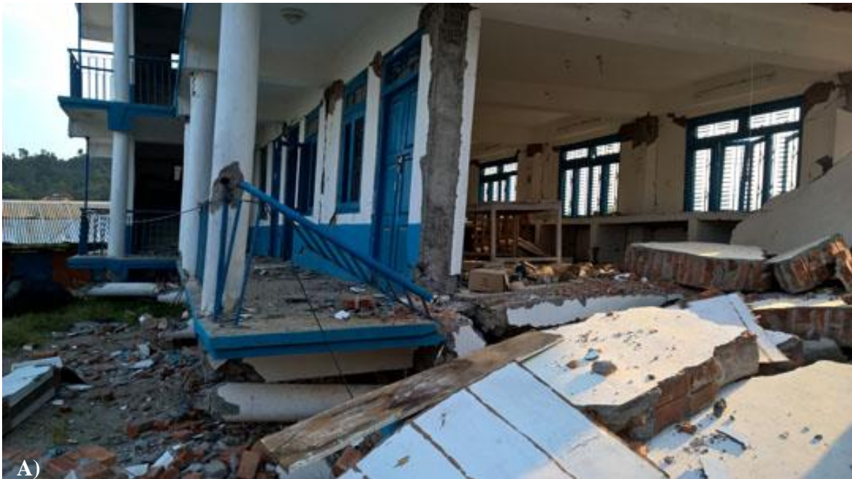
Figure 18A, 18B: The ruins of a 4 storey tall school in Sangachowk, Sindhupalchowk. The ground floor has collapsed completely! The headmaster told us that, had it been a school day, they could have lost upto 400 children!!
