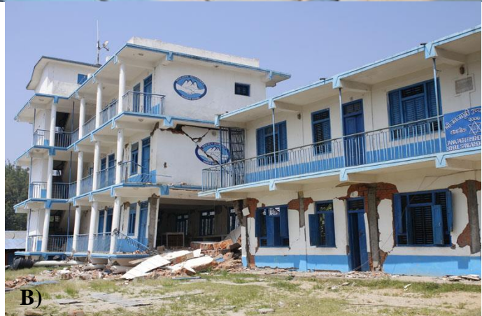
Figure 18A, 18B: The ruins of a 4 storey tall school in Sangachowk, Sindhupalchowk. The ground floor has collapsed completely! The headmaster told us that, had it been a school day, they could have lost upto 400 children!!
