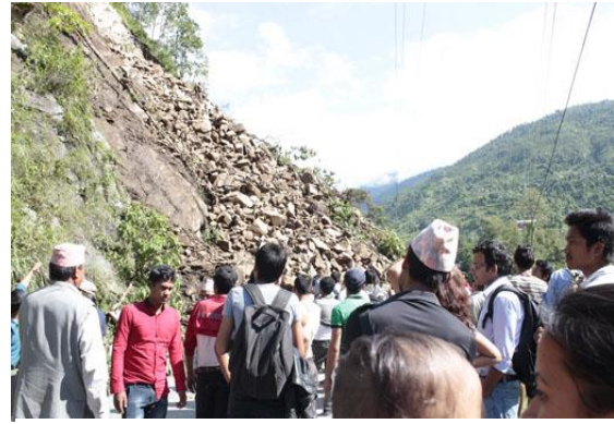
Figure15: Difficult logistics: Road block due to landslides at Balefi
